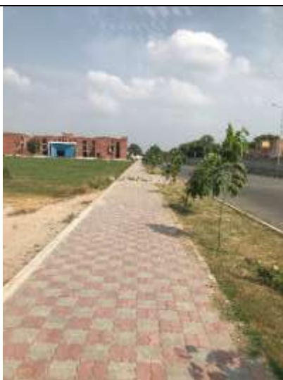
Pedestrian Footpath (Air university, Multan Campus)
