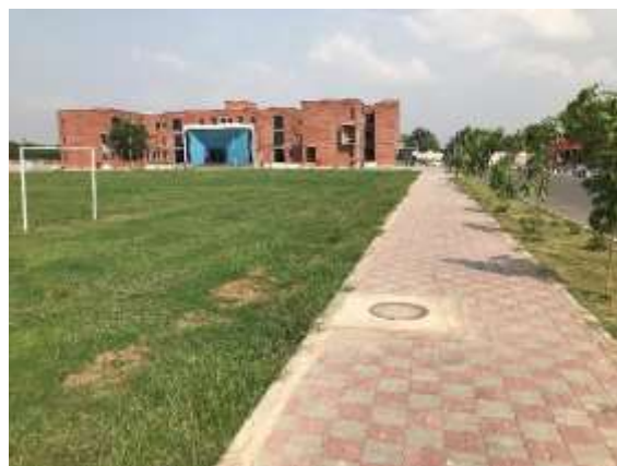
Pedestrian Footpath (Air university, Multan Campus)
